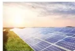
Energy Storage System
